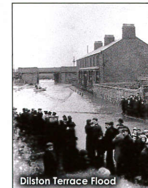
Dilston Terrace Flood
